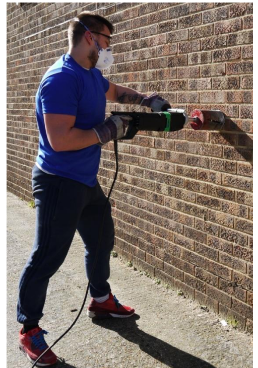
CORRECT DRILLING POSITION
